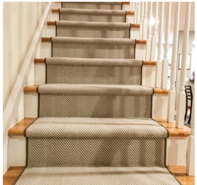
Example of Hollywood Finish on Stairs
