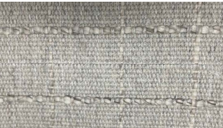
Acceptable seam for looped carpet
