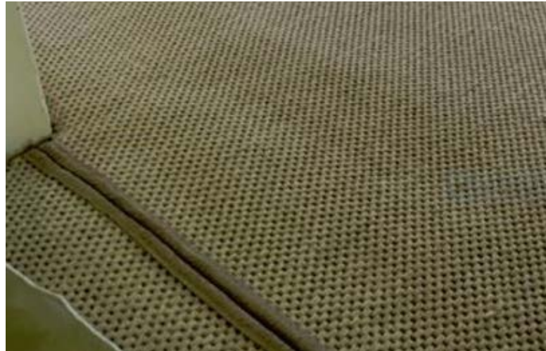
Example of a serged seam on a flat-woven carpet
